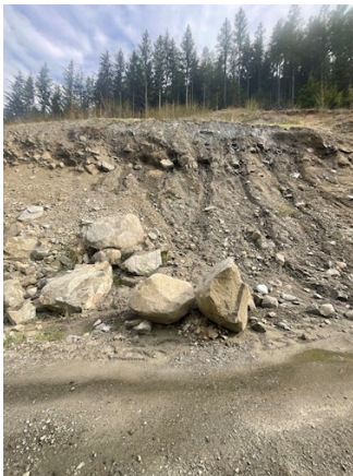
Upslope rock debris
